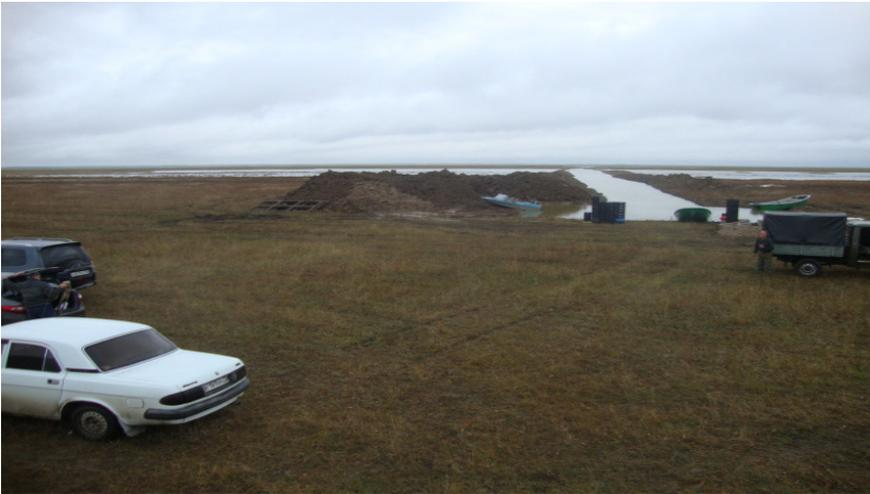
*Fig.2. The melioration channel (in open water — for the movement of watercraft; in winter — for the installation of turbo aerators and the capture of whitefish that remain in the process of fishing “in open water”*
